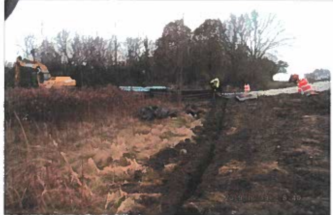
20191119KKJ Trenching in silt fence .JPG
