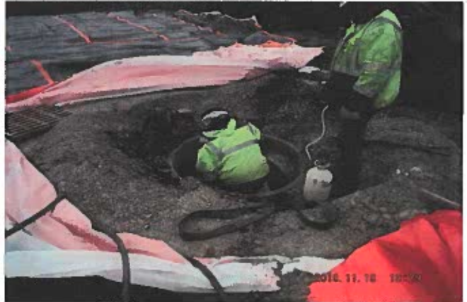
20191119KKJ Trimming structure 11 .JPG
