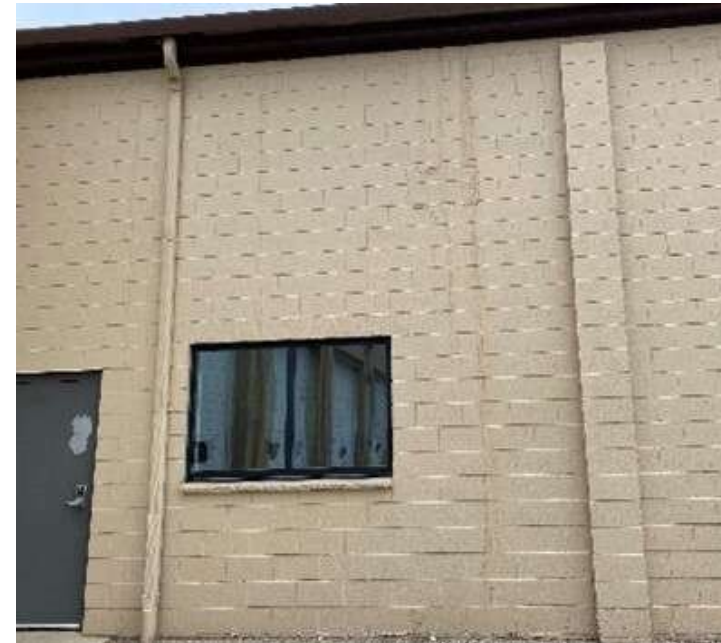
Roof Leaks - Repair
