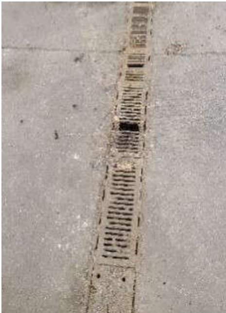
Trench Drains - Replace
