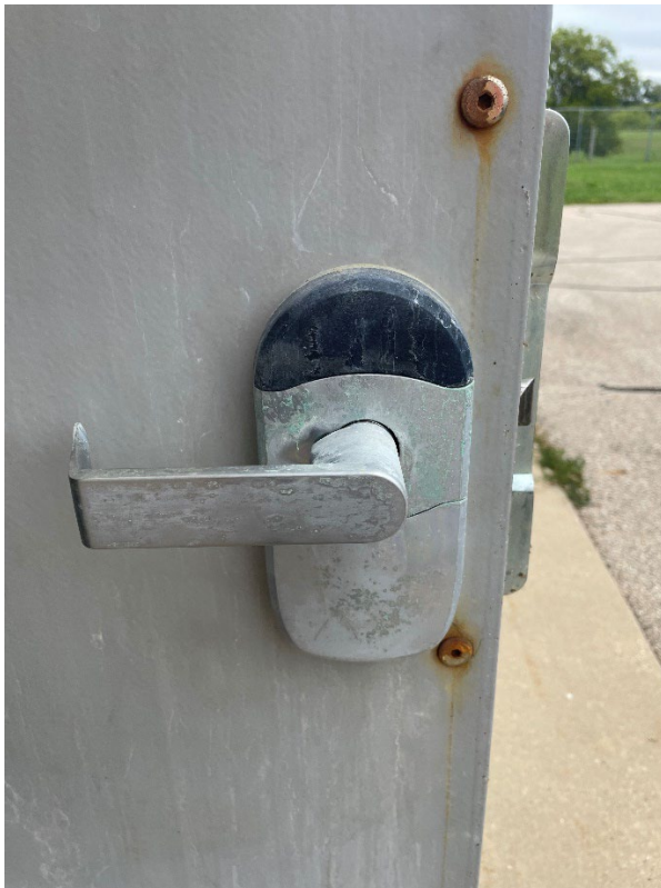
Photo 1, Doorknob exposed to fluoride
