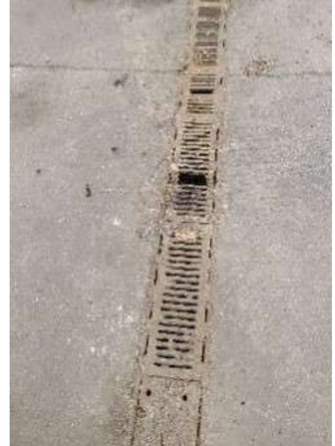
Trench Drains - Replace
