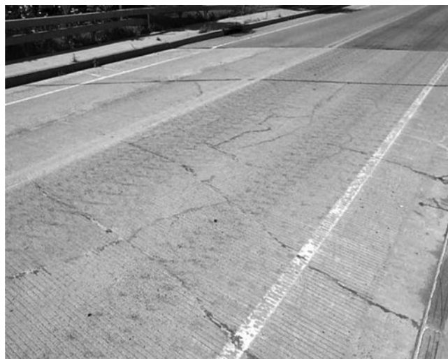
Fig. 1—Methacrylate flood coats are well-suited to concrete slabs that have a large number of random cracks but no evidence of steel corrosion or AAR.
