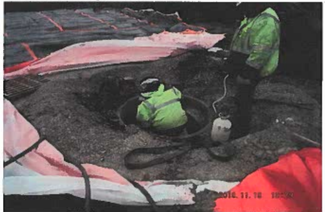
20191119KKJ Trimming structure 11 .JPG
