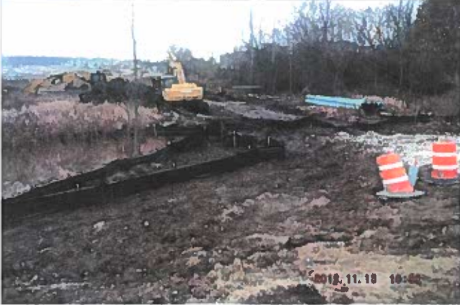
20191119KKJ Silt fence around tracking pad area .JPG
