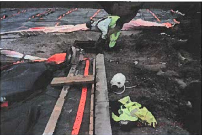
20191119KKJ CB 11 in alignment with curb .JPG
