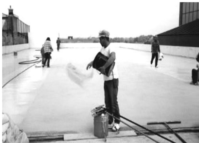
Fig. 3—Aggregate broadcast onto the surface before the resin cures can increase traction.
